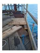
This a reminder that scaffold boards should be secured as soon as they are set, before they are used for a walking/working surface, and no worker should step onto an unsecured board.
