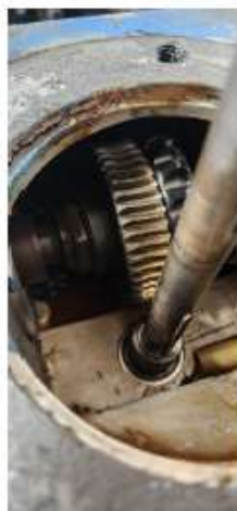
Image of bronze gear in good condition
