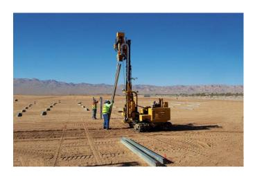
In this particular incident, the pile was lifted and while suspended by the magnet, the metal I-beam pile fell unexpectedly when the magnet detached suddenly. This dropped object is being classified as a serious incident because personnel were in the immediate vicinity
