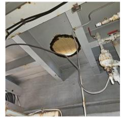
Corrosion over time led to the tabs holding the cover in place to let go, causing it to fall through to the deck below. Fortunately, it did not hit anyone or cause any damage. A black plastic containment berm had been placed over the hole and a cutting bow was landed near it. When a worker walked next to the cutting box, where the hole was hidden by the berm, the tabs welded to the insert cover let go, causing the worker's foot to go about 6 inches deep.
