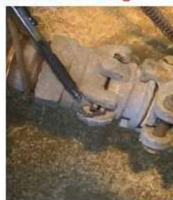
Bailing wire used by paint crew on different fitting
