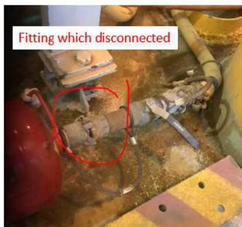
Bailing wire used by paint crew on different fitting
