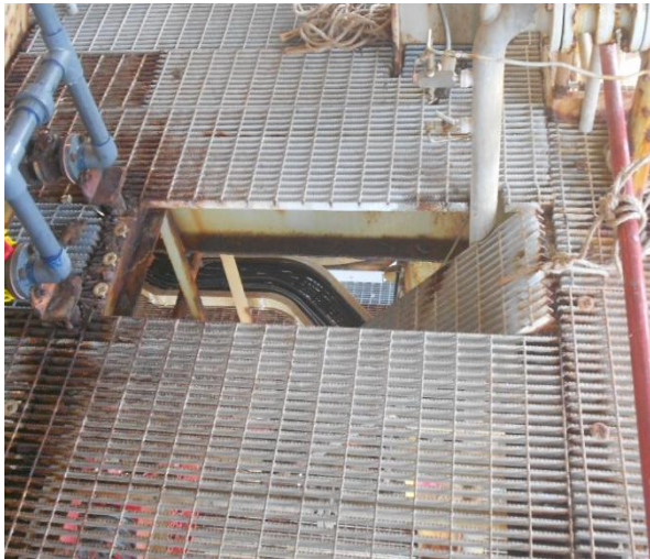
Side view of collapsed grating
