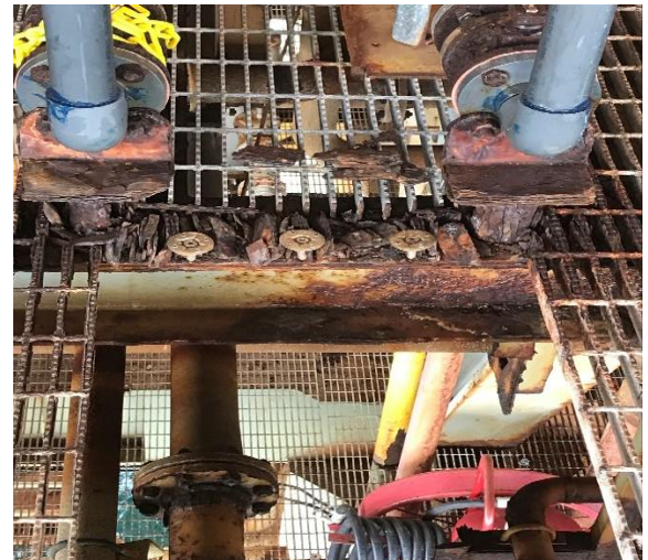
Corroded End of Grating
